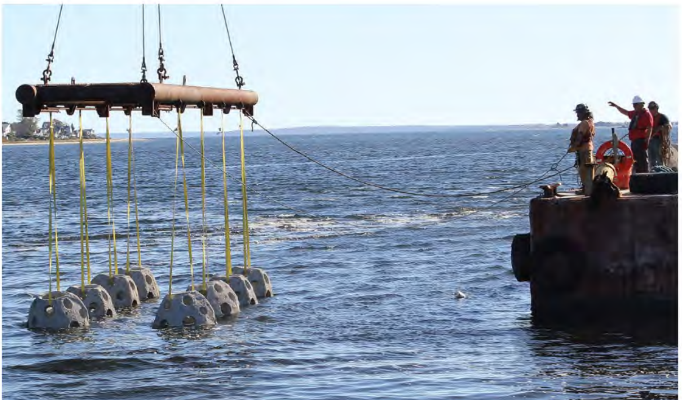
Placing reef balls at Sabin Point in Riverside, Rhode Island.
