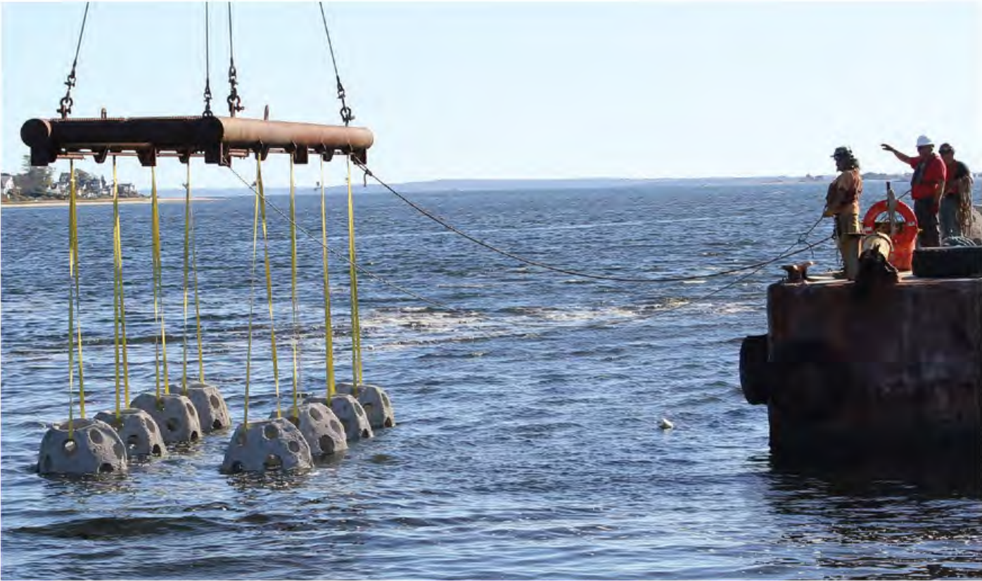
Placing reef balls at Sabin Point in Riverside, Rhode Island. © Timothy Mooney/TNC
