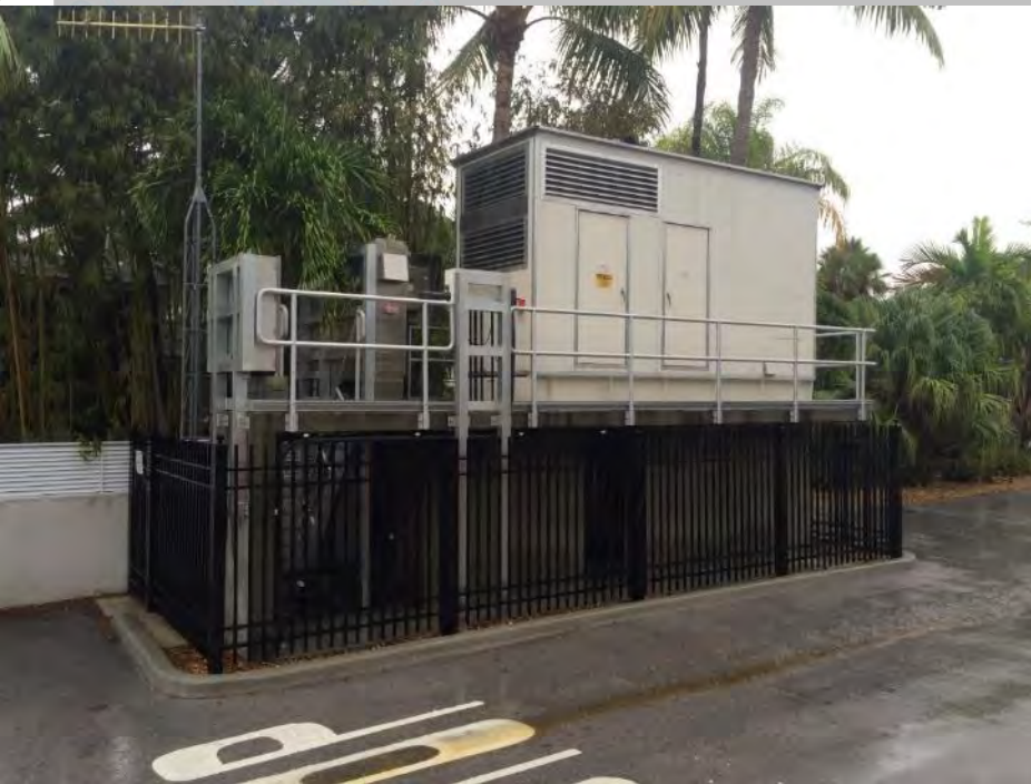
Elevated injection pump station: Key West
